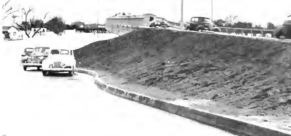
Old section of U. S. 40 across American River overflow was flooded but 16th Street Viaduct opened Sept. 14, 1942, carried all traffic
